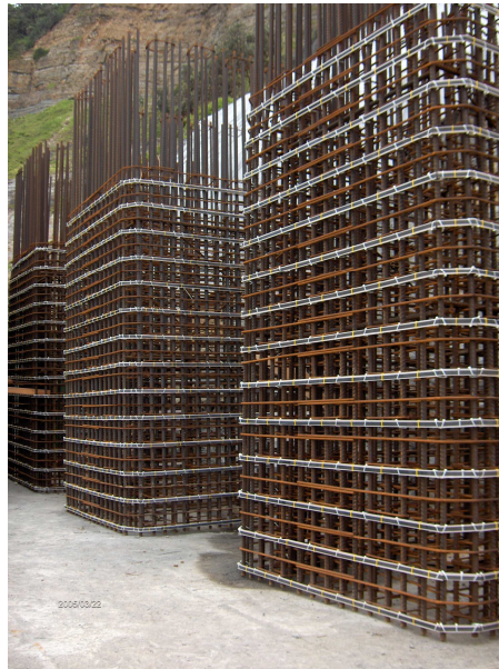
Figure 7: Anode installation on column steel reinforcement cages
