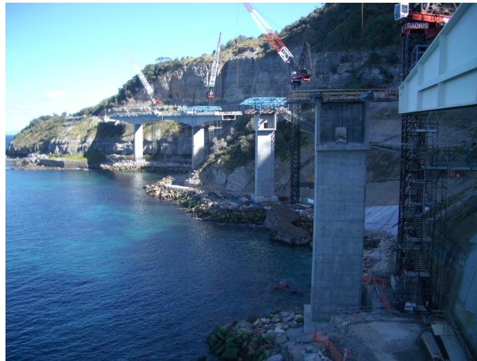
Figure 2: Sea Cliff Bridge during construction. CPrev applied to pier columns and pilecaps
